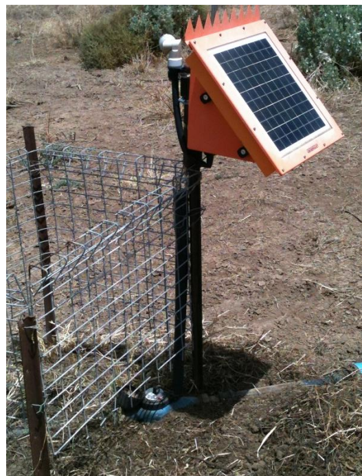
The remote water monitoring system is powered by solar panels
