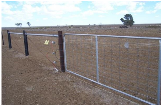
The electric fence design is six plain wires with a barb on top.
