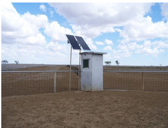
The single Gallagher 2800i Solar Energiser is located at the centre of the fence line.
