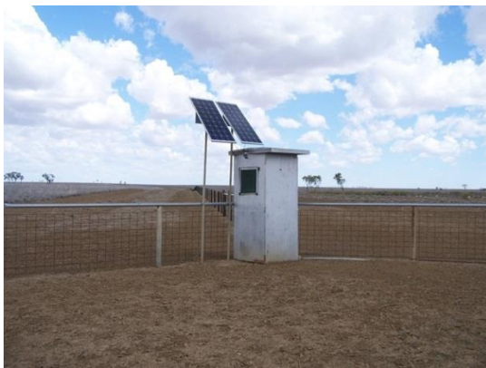
The single Gallagher 2800i Solar Energiser is located at the centre of the fence line.
