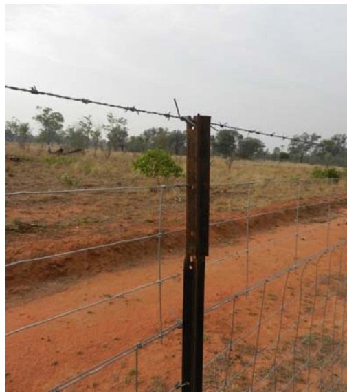
Photo 7: Fence 3 – additional height added to the fence
