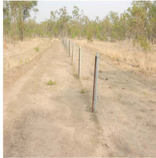
Photo 1: Fence 1 – total height of fence is 125cm
