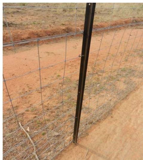
Photo 15: 15cm gaps between vertical wires were more effective than 30cm gaps
