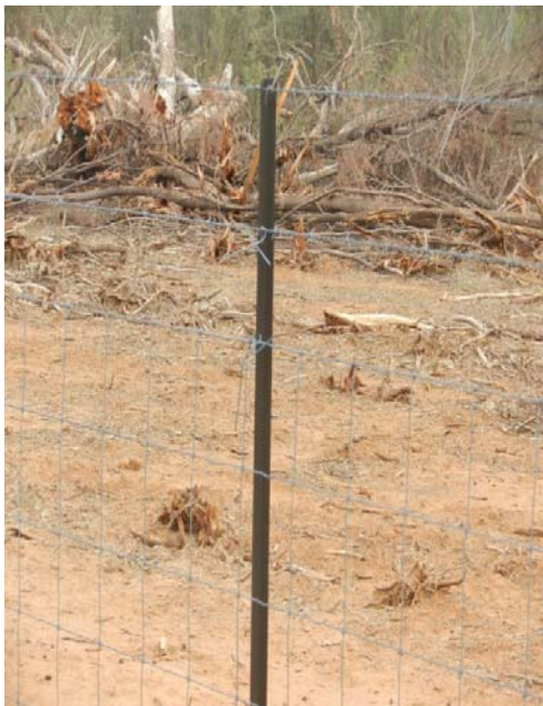
Photo 5: Fence 2 - 2 barbed wires at the top
