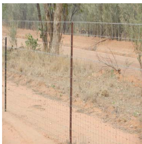
Photo 8: Fence 3 – total height is 160cm high
