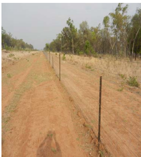
Photo 14: Small posts from existing fence were left and used
