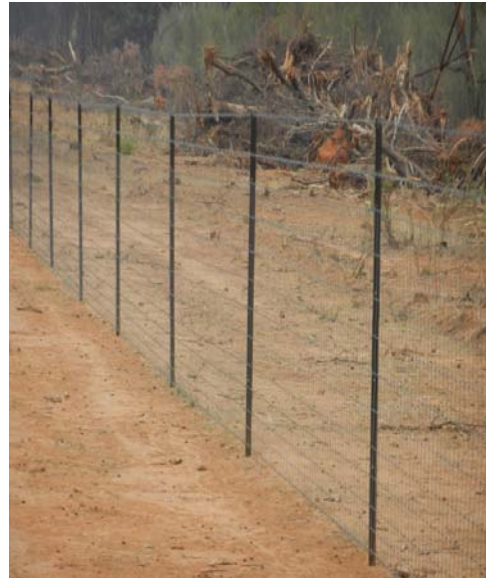
Photo 4: Fence 2 – total height of fence is 135cm
