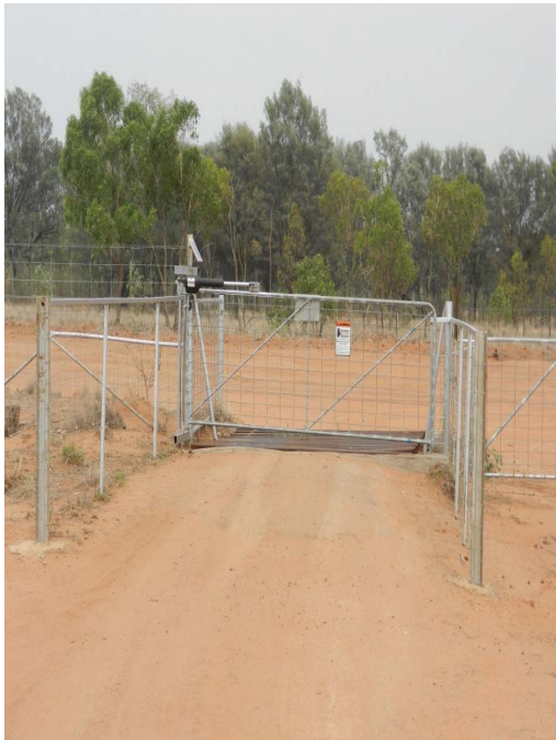
Photo 12: An automatic gate was installed on the driveway grid
