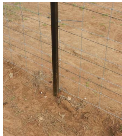
Photo 3: Fence 1 - Existing plain wires were left to help strengthen the fence
