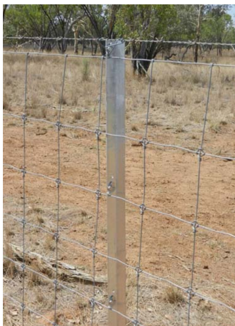
Photo 7: Fence 2 – 1 barbed wire at the top of the fence
