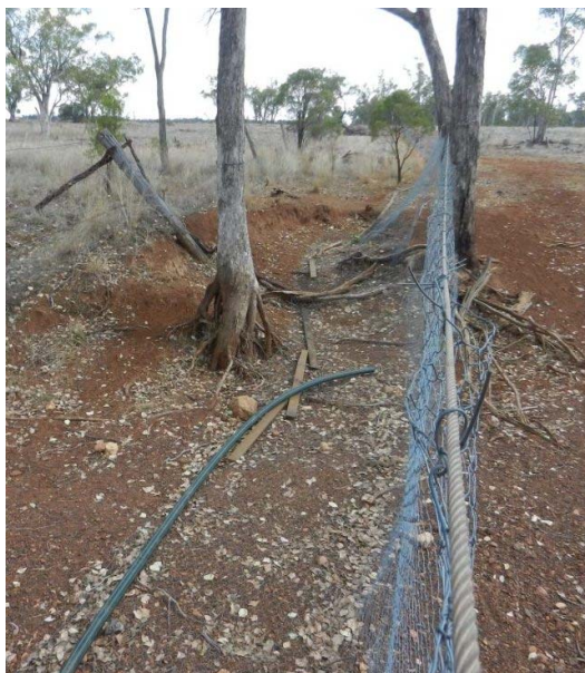
Photo 12: The netting is left long to overhang along the ground to stop animals getting through after flooding
