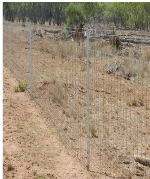
Photo 6: Fence 2 – Total height of the fence is 150cm
