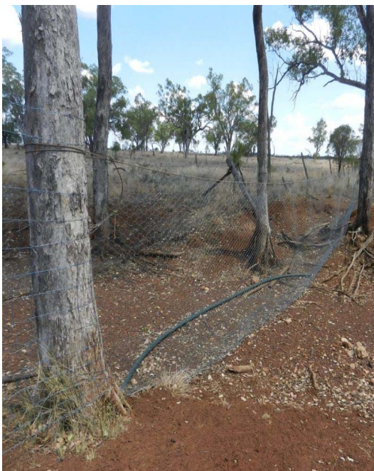
Photo 10: Cable was suspended between 2 trees and the netting was tied to the cable
