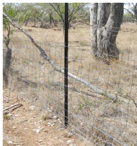
Photo 5: Fence 1 - A plain wire was run along the bottom of the fence for extra strength
